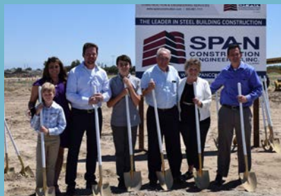
The Ueland family, owners of TranPak, breaking ground at their new 65,000 square foot manufacturing facility.
